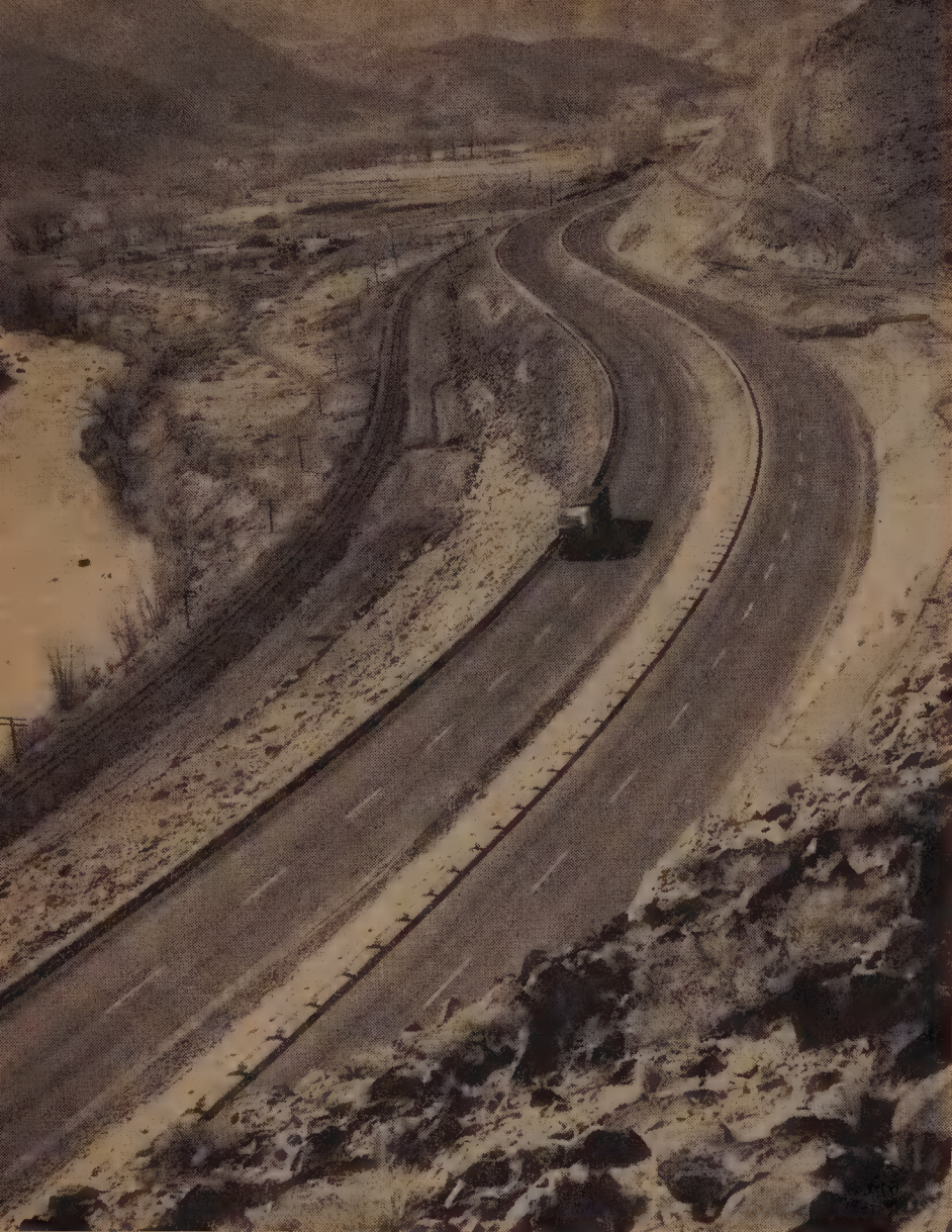
This divided section of Highway 40 in Truckee River Canyon east of Sparks is typical of modern Nevada road construction.
